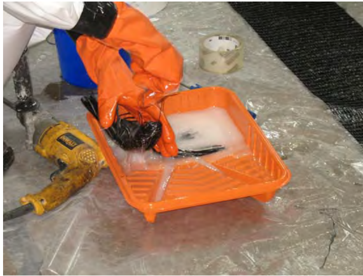
Figure D.16 Saturation of CFRP anchor with epoxy
