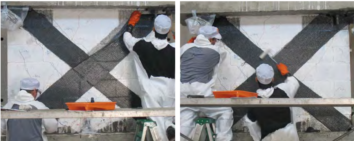
Figure 6.54 Application of the 12in.wide CFRP strip (left) and second 9in.wide CFRP strip (right) later.
