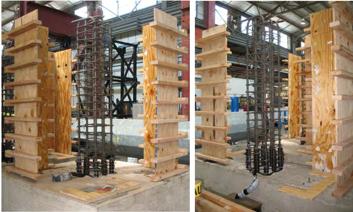
Figure 5.92 Internal reinforcement and formwork for each specimen
