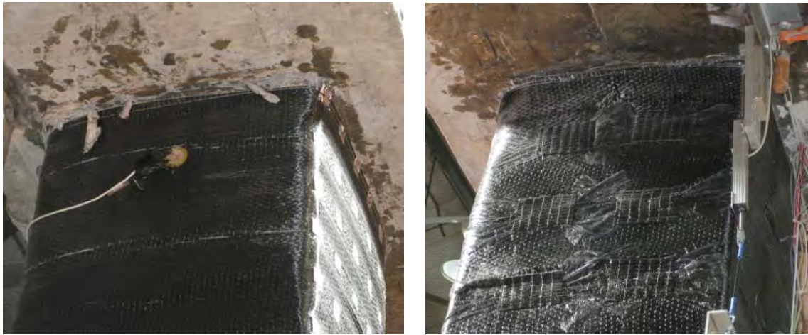
Figure 5.74 Good condition of CFRP sheets and anchors after the 9 th hysteretic cycle
