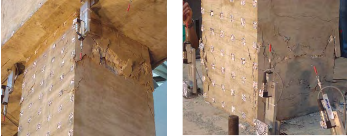
Figure 5.27 Top(left) and bottom (right) of the column. Cracks and some spalling of cover are observed on both extremes of the column.
