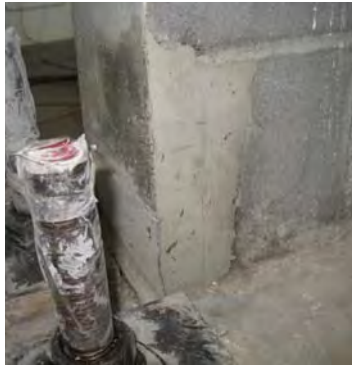
Figure 6.40 Repair mortar to fill the damaged south corner of the wall
