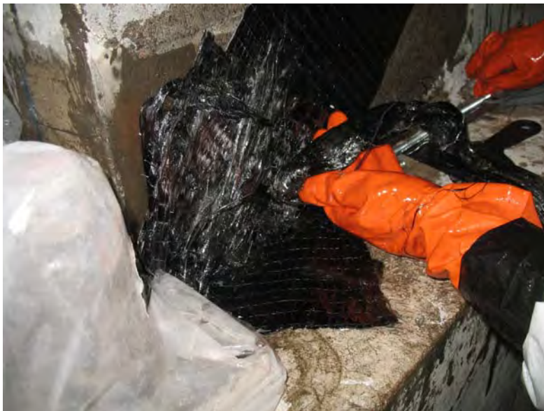
Figure D.19 Installation of CFRP anchor
