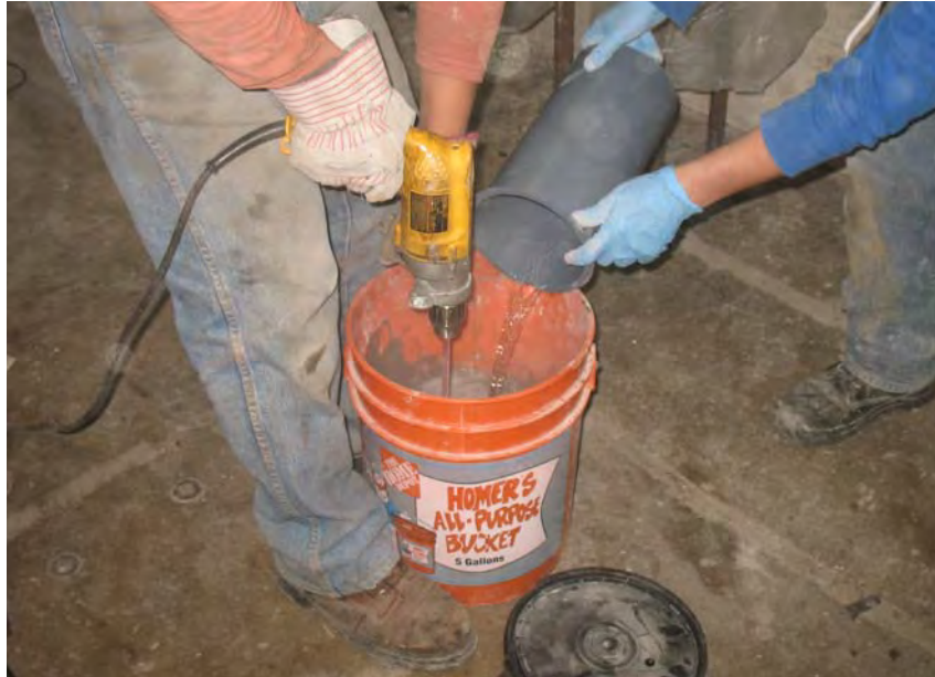
Figure B.3 . Mixing repair mortar with water to apply on the damage top of column
