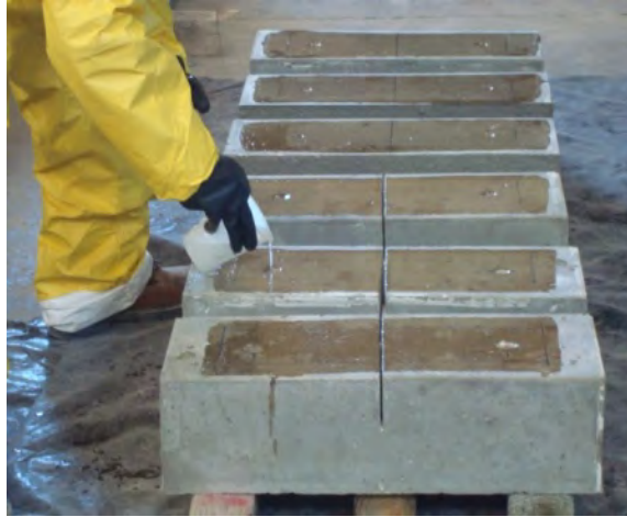
Figure 4.25 Application of the epoxy into drilled holes for CFRP anchor.
