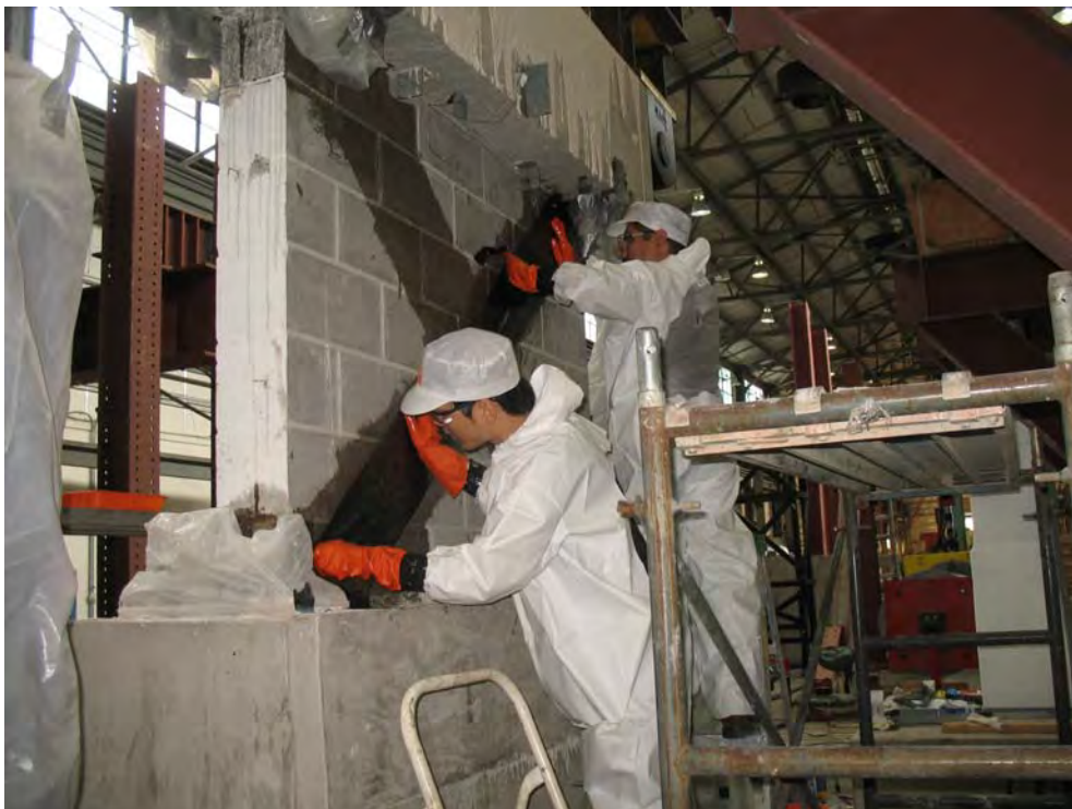
Figure D.15 Application of CFRP strip on back side
