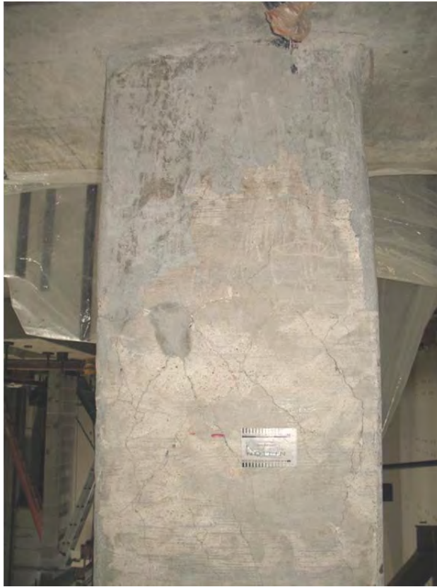
Figure B.5 Condition of the top of column after the mortar dried
