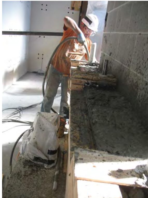
Figure D.5 Placement of the concrete ring
