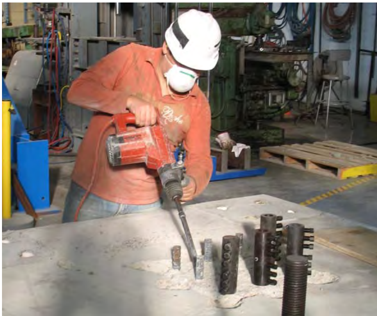
Figure C.3 Removing concrete for installation of mechanical couplers
