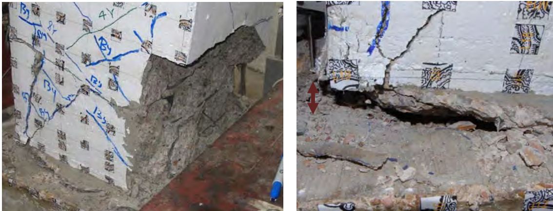
Figure 5.134 Close-up view of the column base. Exposed mechanical splices under compression stress at south face (left) and lifting on the north face (right)
