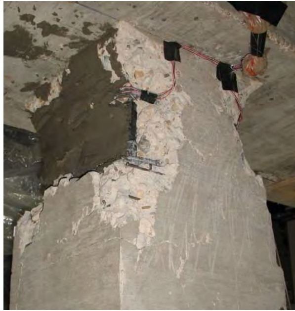
Figure 5.43 Application of repair mortar and CFRP at top
