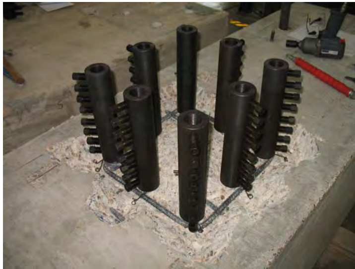
Figure 5.88 Long mechanical splices placed on protruding bars
