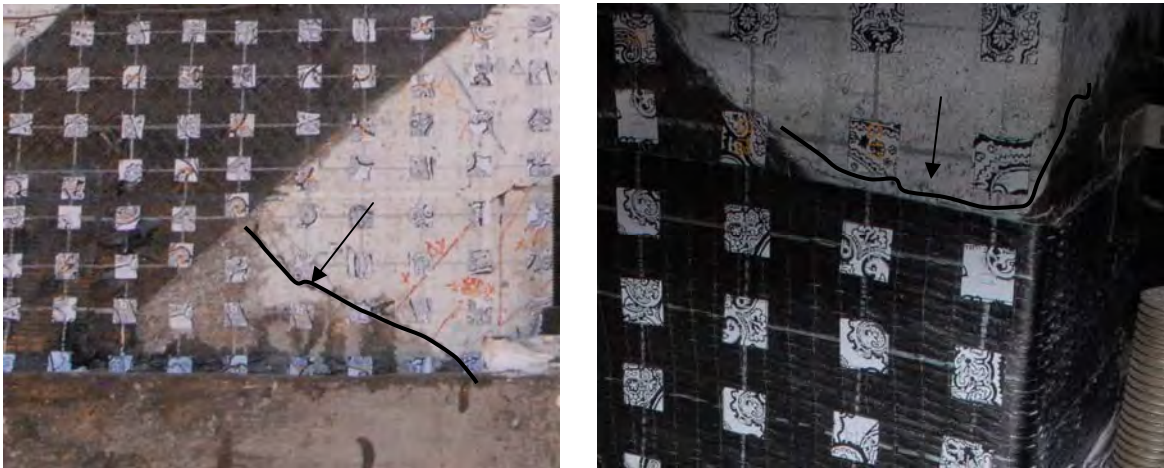
Figure 6.69 Existing cracks opened after reach maximum south (left) and north (right) lateral displacement
