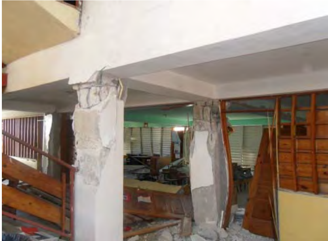
Figure 1.1 Weak Column Strong Beam Join. Haiti Earthquake – 2010 Mag. 7.0
