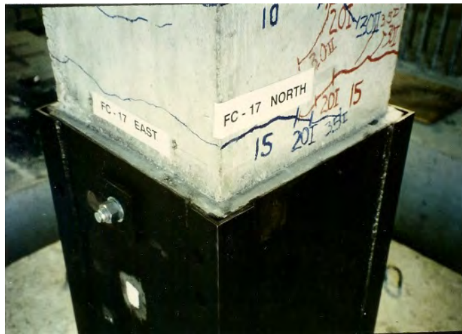
Figure 2.6 View of the retrofitted column after the test (Aboutaha, 1994)
