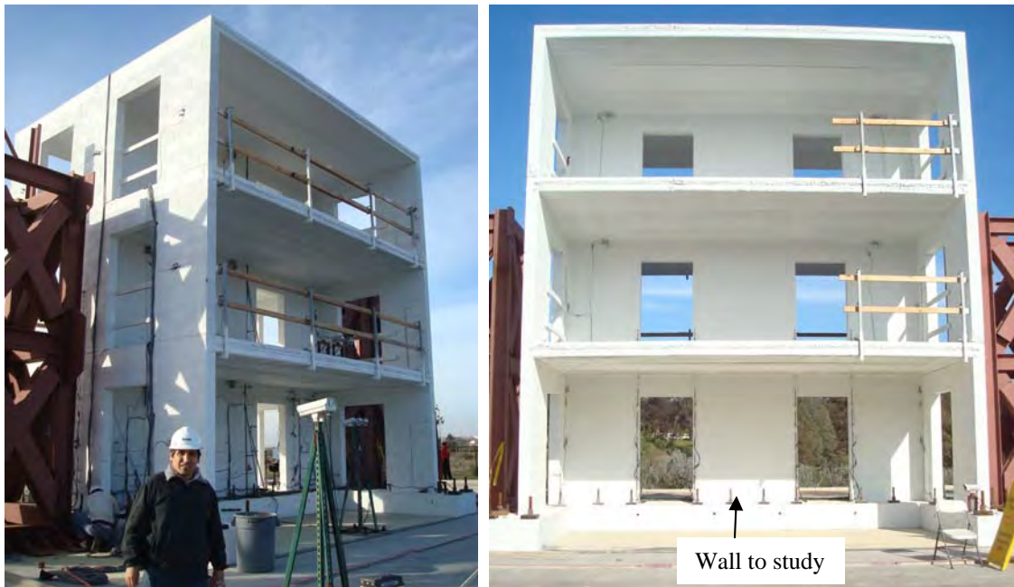
Figure 6.1 Full-Scale three-story reinforced masonry structure. Side and elevation view.
