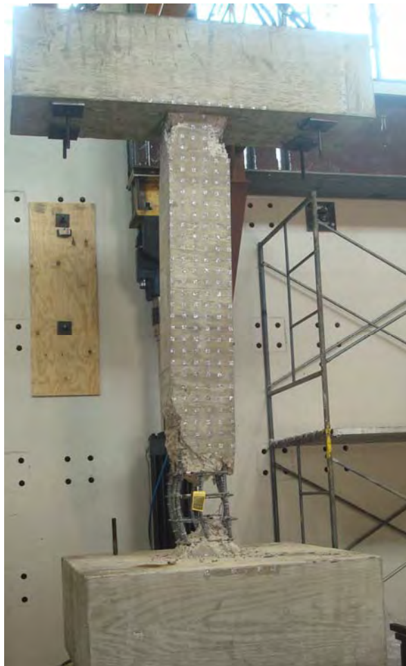
Figure 5.36 Condition of column prior to retrofitting
