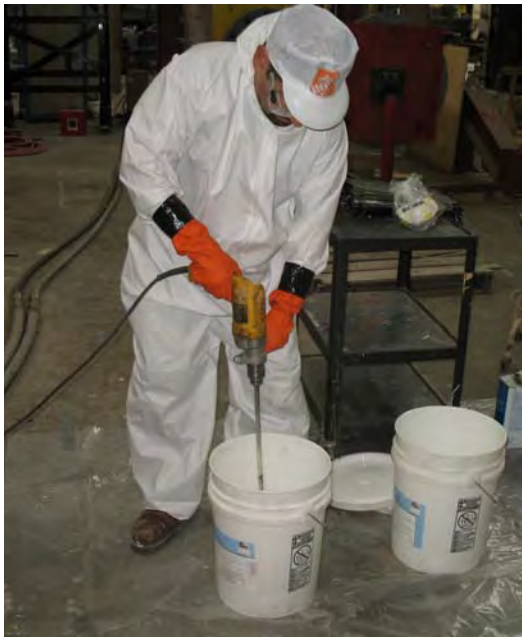
Figure D.11 Mixing components to prepare epoxy for CFRP application
