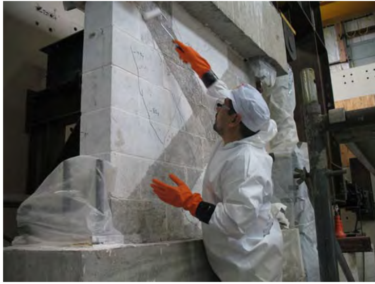
Figure D.12 Application of the epoxy on front surface
