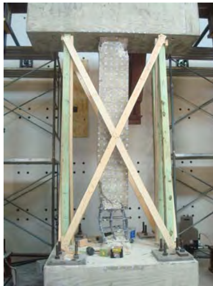
Figure B.1 Severely damaged column RC-1 removed from the test setup
