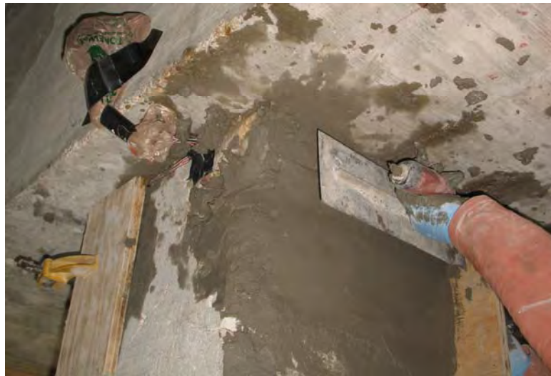
Figure B.4 Application of the mortar on the column replacing the cover
