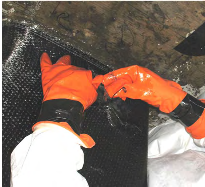
Figure 5.46 Application of the CFRP anchors.
