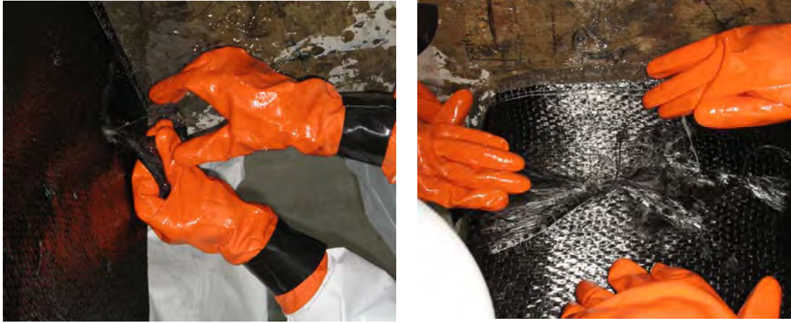
Figure B.10 Application of the CFRP anchor (left) and spreading the fan on the surface (right)
