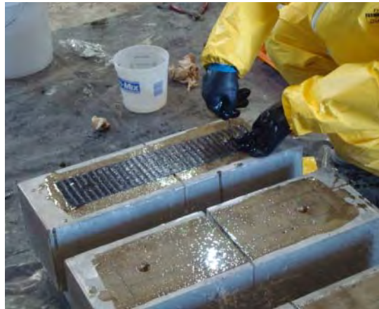
Figure 4.27 -- Installation of CFRP anchor in concrete beam.
