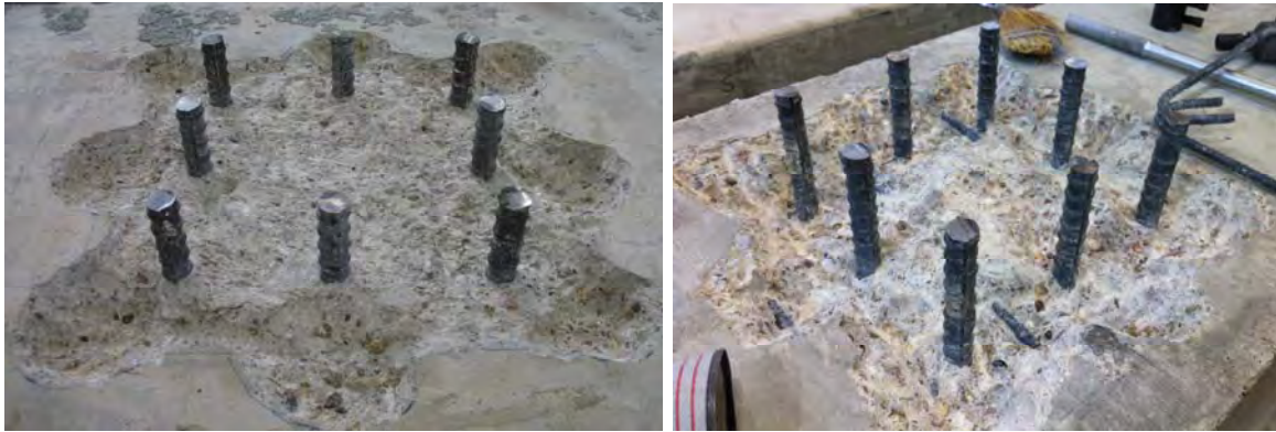
Figure C.4 Protruding bars prior to installation of short splices (left) and long splices (right)
