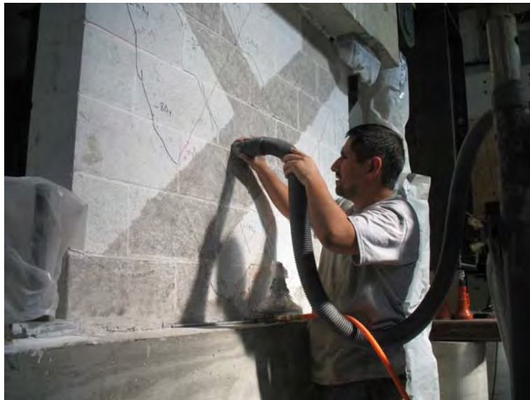
Figure D.9 Cleaning the surface prior to application of CFRP sheet
