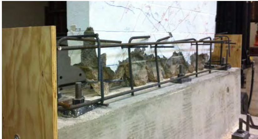
Figure 6.38 Cage of the concrete ring placed.
