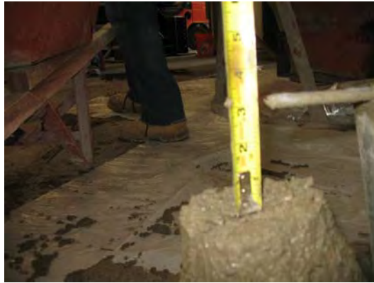
Figure C.10 Concrete placement: slump 3.5in
