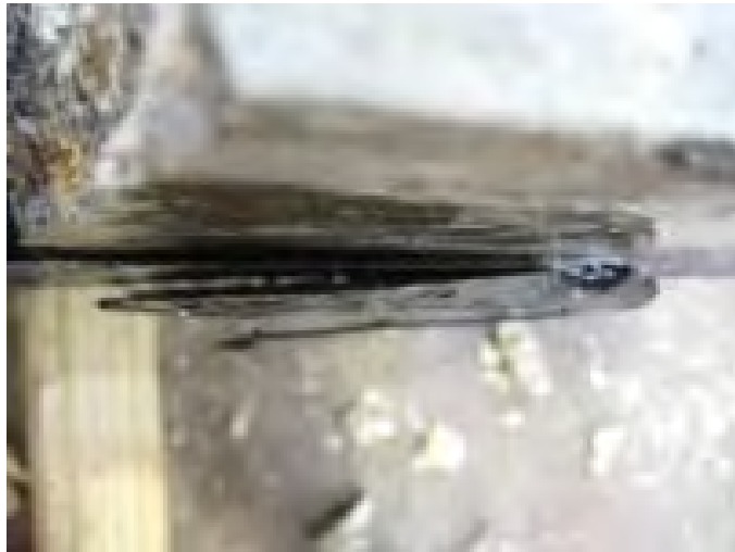
Figure 4.22 Anchor fan debonding due to poor quality epoxy
