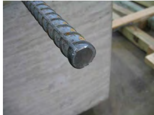
Figure C.6 Grinding of bar end prior to inserting the bar into the splice
