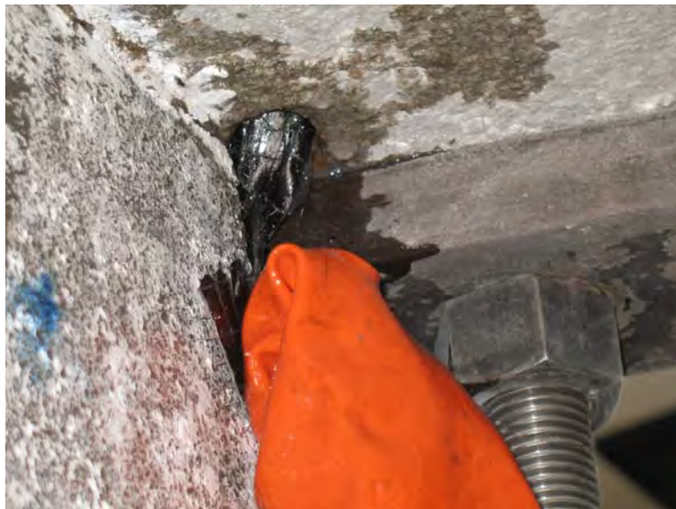
Figure D.17 Insertion of CFRP anchor into the drilled hole
