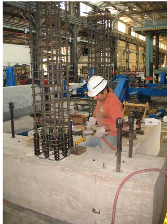
Figure C.7 Tightening of the splice bolts using impact wrench
