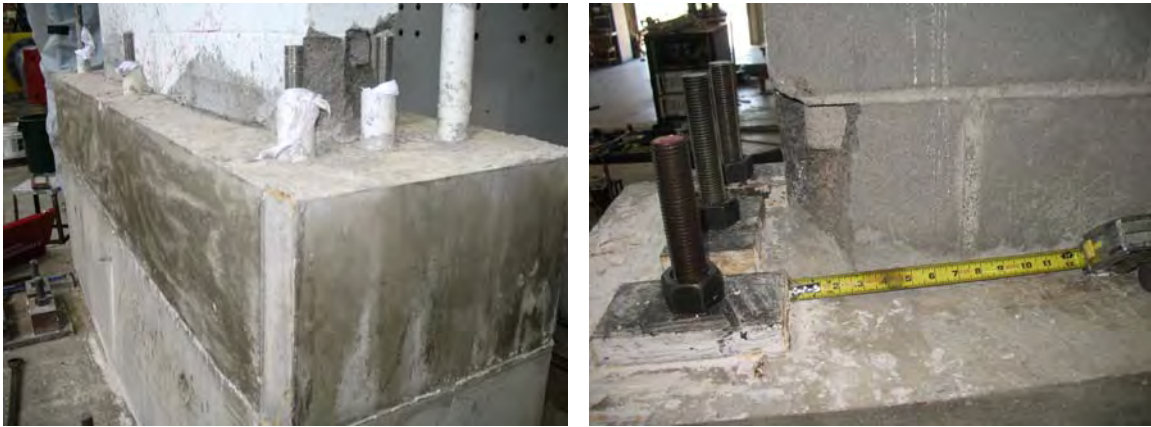
Figure D.6 Concrete ring after removal of form (left) and corner before repair with mortar (right)
