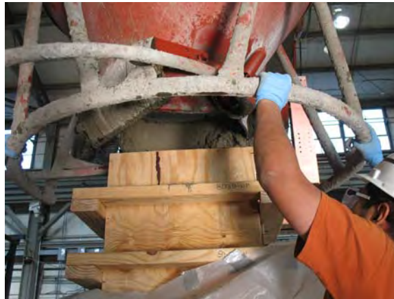
Figure 5.93 Placement the concrete into the formwork
