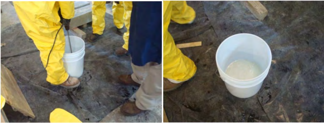
Figure 4.24 Preparation of the epoxy: Mixing of the epoxy component (left) and Epoxy ready to use (right)
