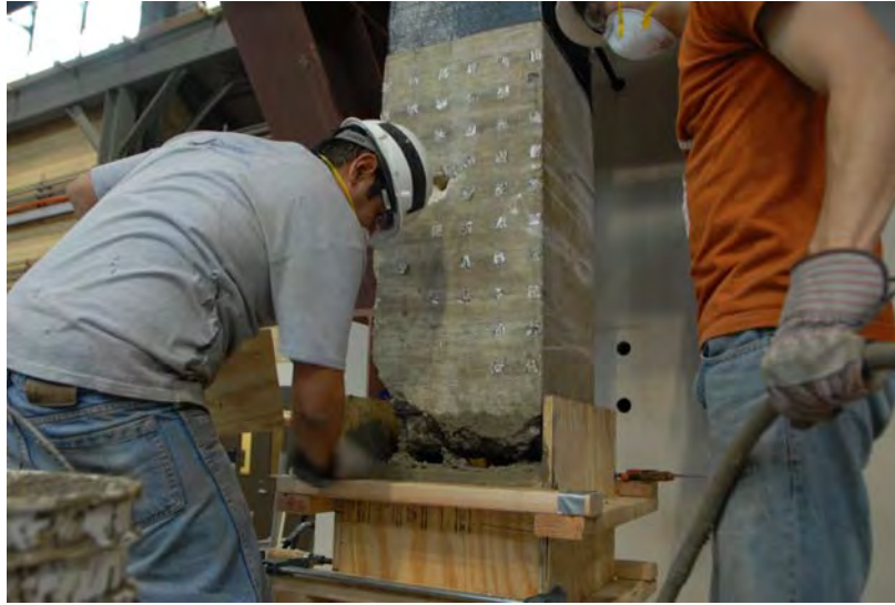
Figure B.19 Placing of concrete in form
