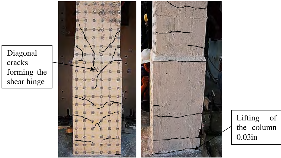
Figure 5.65 Crack pattern appeared at 1.6in lateral deformation (1.43% drift ratio)
