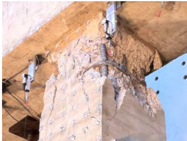
Figure 5.29 Concrete crushed, buckled longitudinal bars in the top of column
