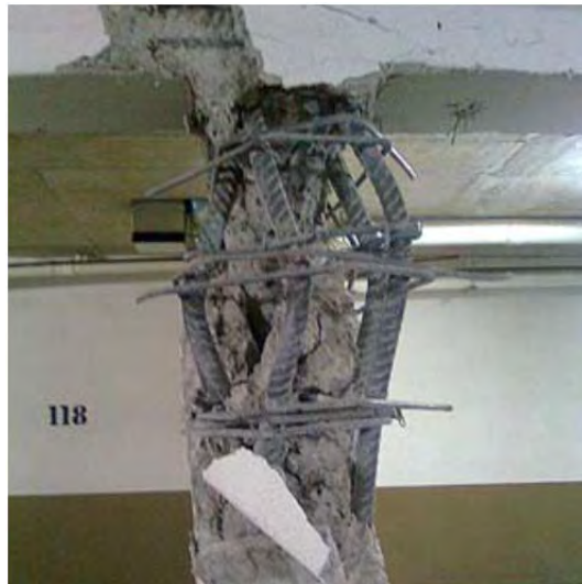
Figure 1.2 Deficient Shear Reinforcement at Reinforced Concrete Columns Chile Earthquake – 2010 Mag. 8.8
