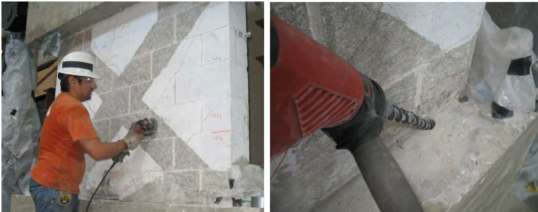
Figure 6.52 Drilling of the surface (left) and the holes (right)
