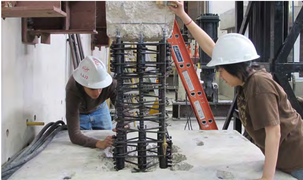
Figure B.15 New bars applied together with the splices
