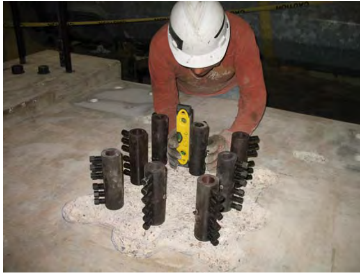
Figure 5.87 Short mechanical splices placed on protruding bars
