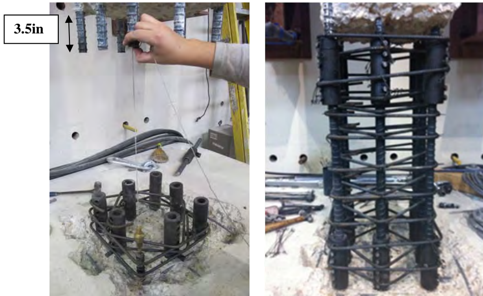
Figure 5.48 Installation of replacement bars using the Short Mechanical Splices
