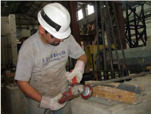
Figure C.6 Grinding of bar end prior to inserting the bar into the splice
