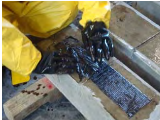
Figure 4.28 -- Spreading out of the CFRP anchor fan.
