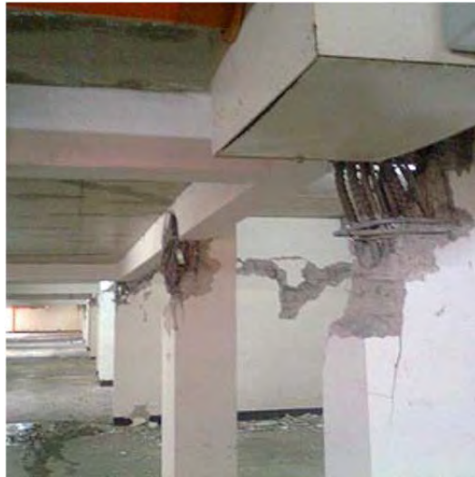
Figure 1.3 Deficient Shear Reinforcement in Columns and Walls Chile Earthquake – 2010 Mag. 8.8
