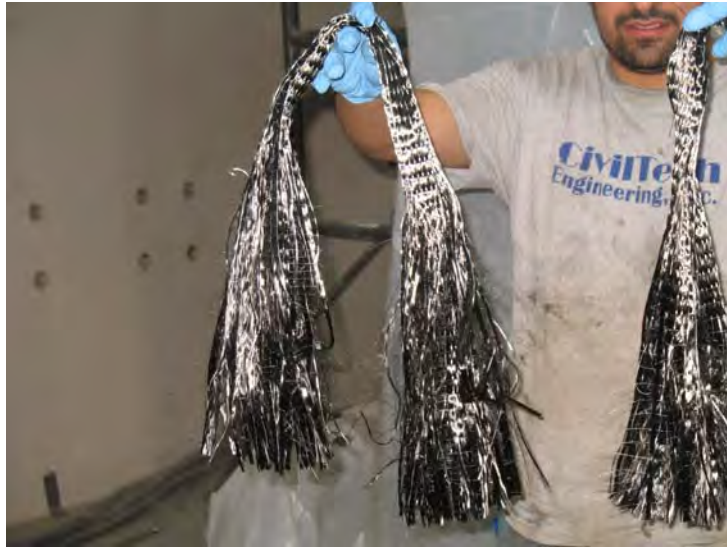
Figure D.10 CFRP anchors for the bottom corners
