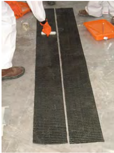
Figure D.14 Application of the epoxy on CFRP strips
