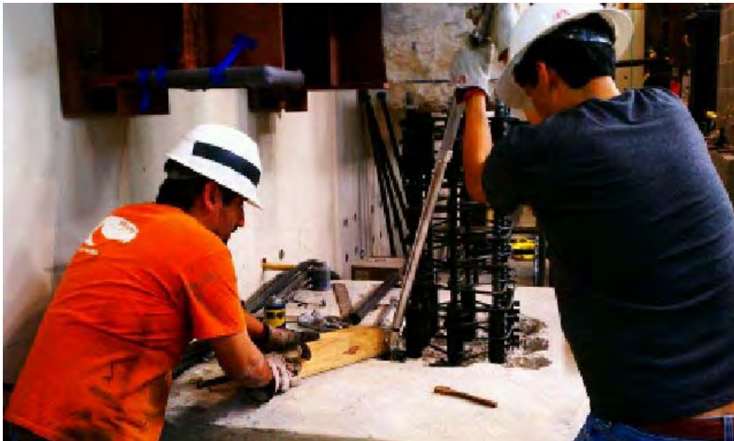
Figure B.16 Tightening of the bottom bolts of splices using ratchet wrench
