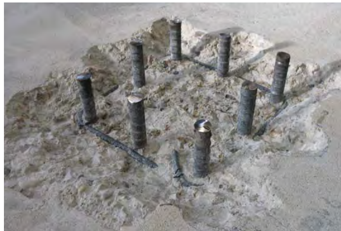
Figure B.13 Protruded bars to installation of the splices
