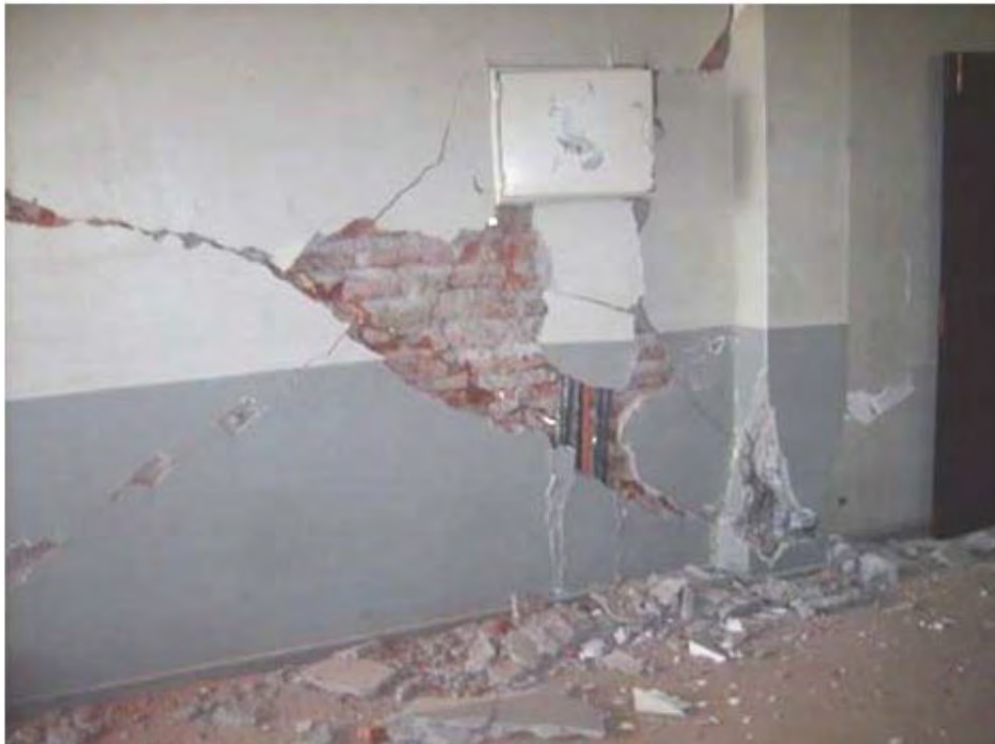
Figure 1.4 Masonry wall with shear cracks. Chile Earthquake – 2010 Mag. 8.8
