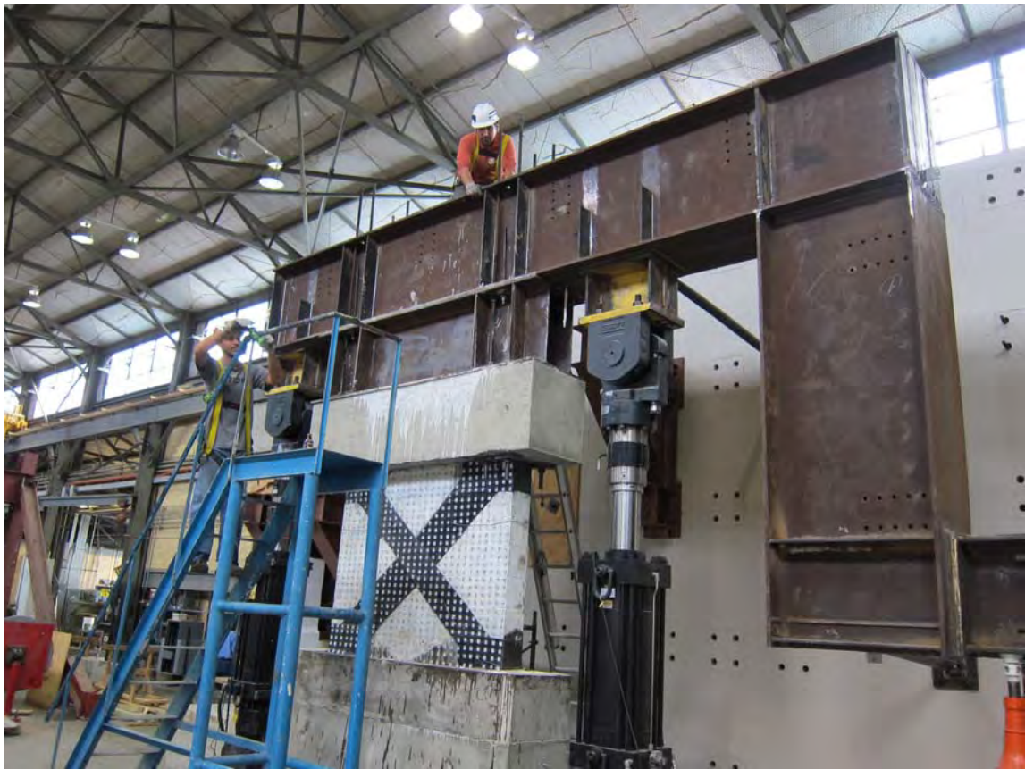
Figure F.5 Installation of rods on RMW-R2 and the L-frame setup
