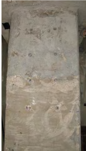
Figure 5.44 Holes drilled for the CFRP anchor installation
