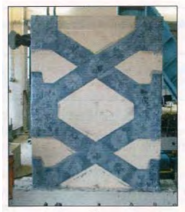
Figure 2.18 CFRP materials applied to the two story frame with infill panels (Pampanin & Akguzel 2011)
