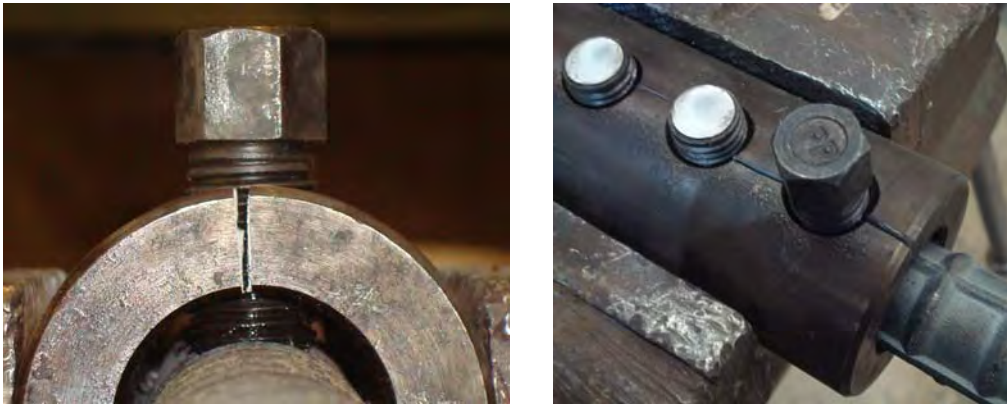
Figure I.1 Crack in coupler after bolt tightening.
