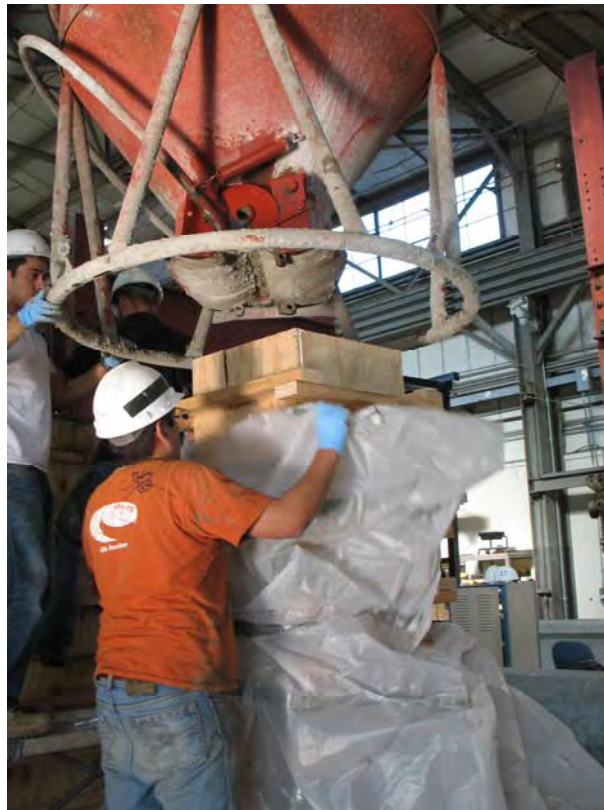
Figure C.11 Placement of concrete in forms
