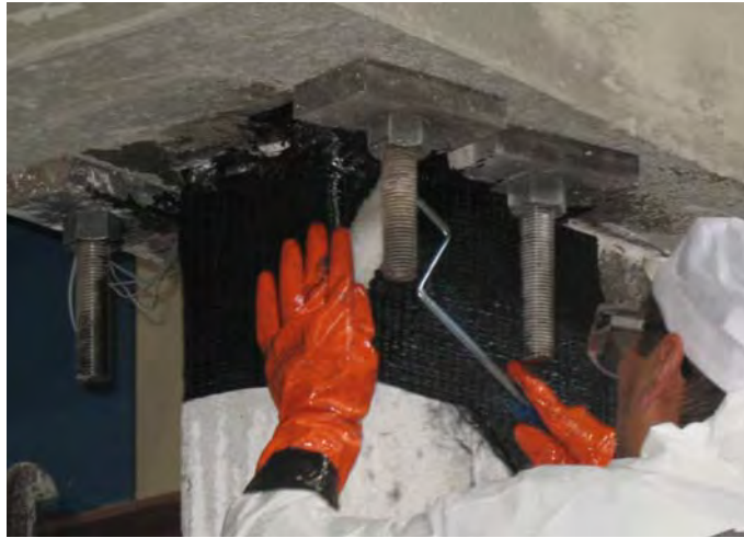
Figure 6.56 Application of the CFRP U-Wrap
