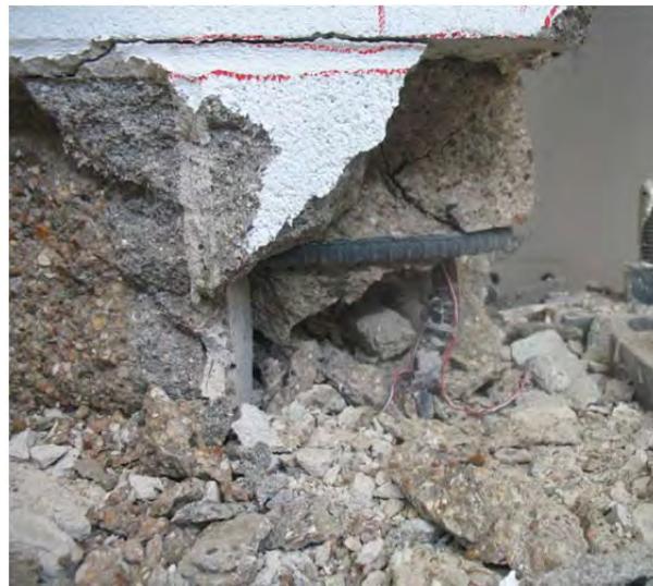
Figure 6.31 Toe crushing of the inferior right corner of the masonry wall.
