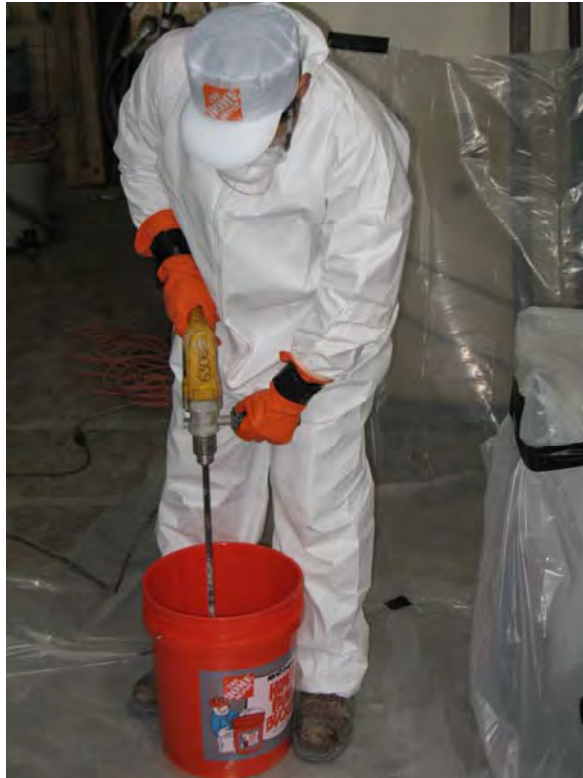
Figure B.6 Mixing epoxy to application of CFRP materials
