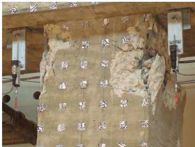
Figure 5.19 Spalling of the cover at top of column.
