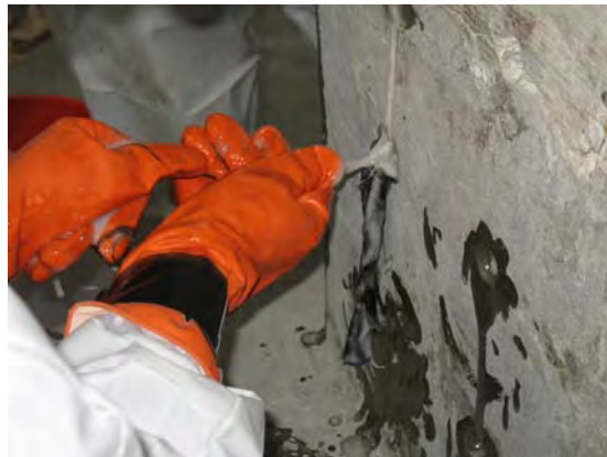
Figure B.7 Application of epoxy into the drilled holes for the CFRP anchors
