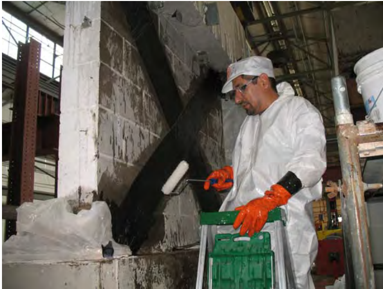
Figure D.18 Saturation of CFRP diagonal strips with epoxy
