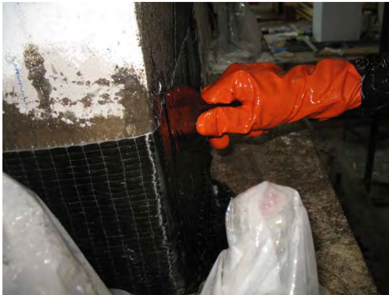
Figure D.21 Application of the CFRP U-patch over the fan anchors
