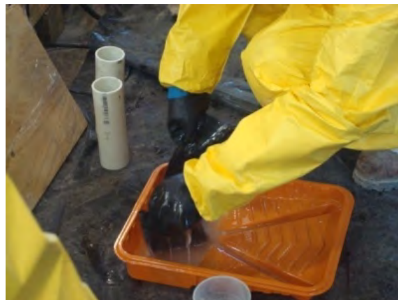
Figure 4.26 Application of epoxy to CFRP materials.
