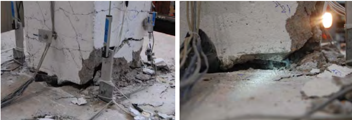
Figure 5.111 Rupture of existing north longitudinal bars loading to south
