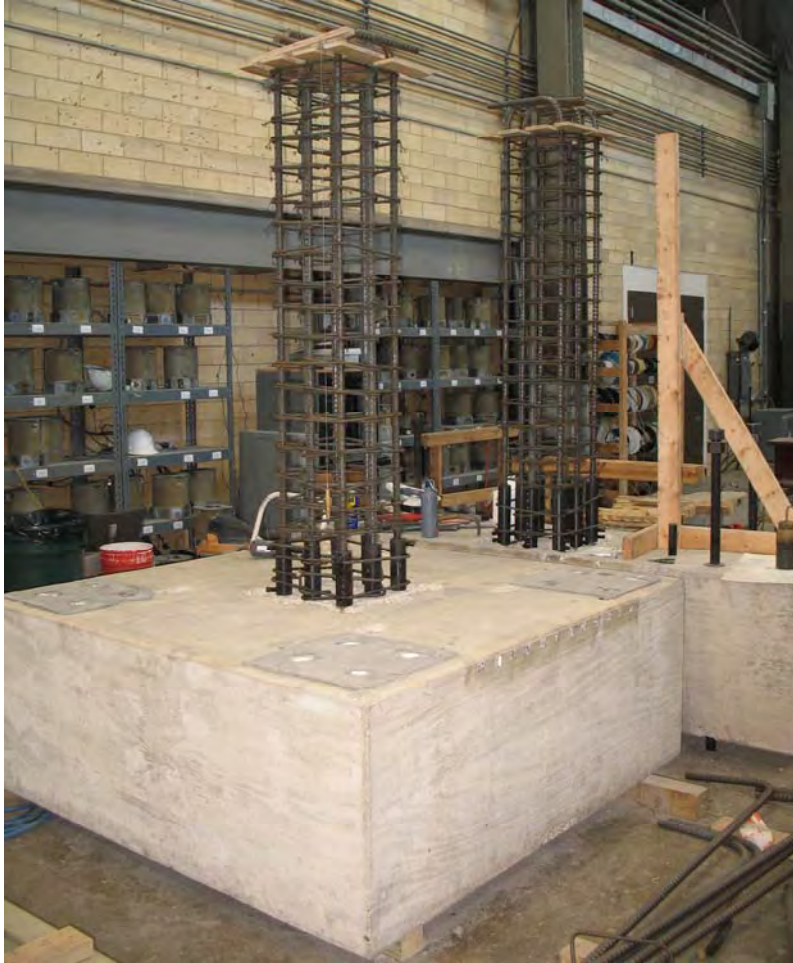
Figure 1.8 New columns connected to existing support with mechanical splices after buckled longitudinal bar removed.
