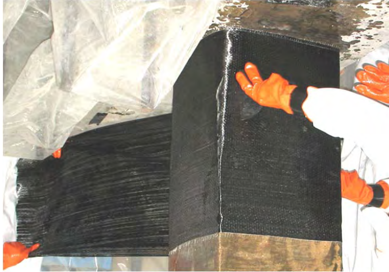
Figure 5.45 Application of the CFRP sheet (jacket) on top of column.
