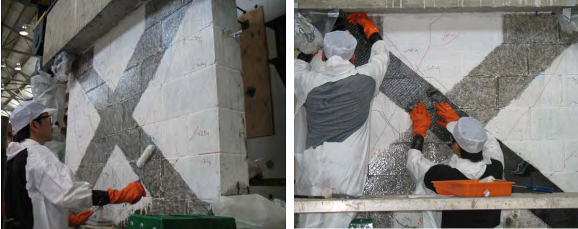
Figure 6.53 Application of epoxy to the surface of the masonry wall (left) and first 9in.wide CFRP strip (right) afterwards
