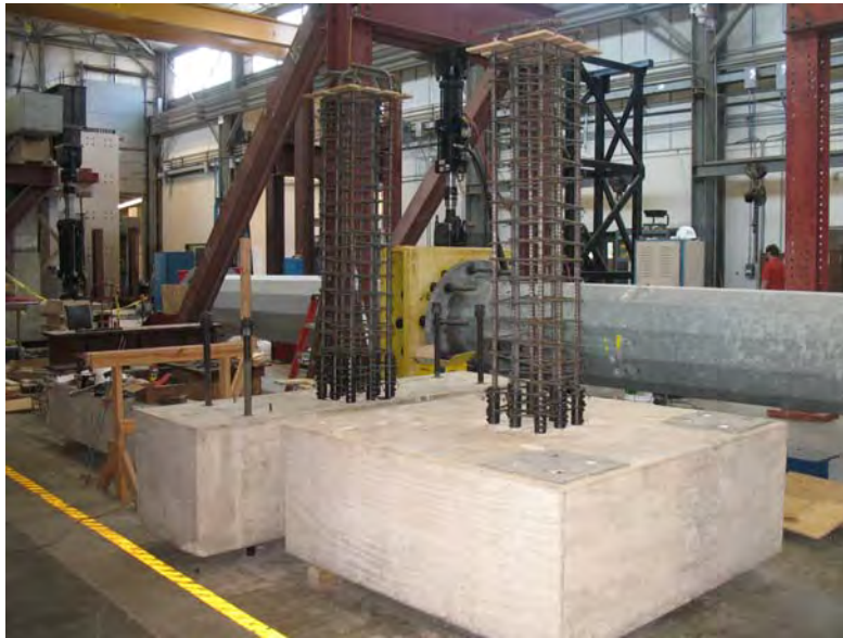
Figure C.8 Reinforcement cages for columns
