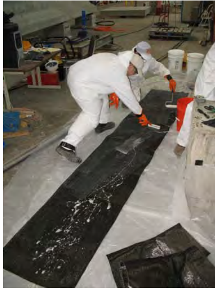
Figure B.8 Saturation of epoxy to the CFRP sheet
