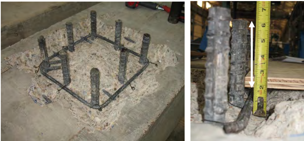
Figure 5.86 Top beam with the existing bar removed for the application of the long mechanical splice
