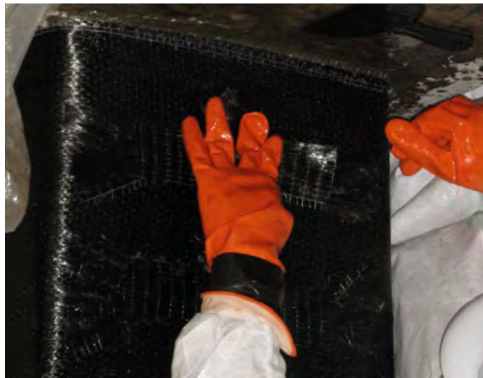
Figure B.11 Application of the CFRP patch on the fans of the anchors
