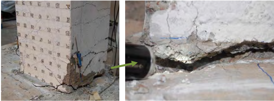
Figure 5.108 Rupture of original south longitudinal bars pushing to north direction.
