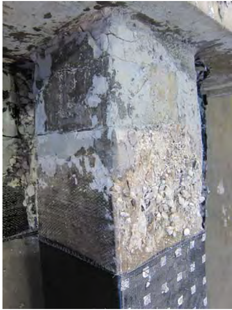
Figure G.7 Condition of top of column after the removing of CFRP jacket
