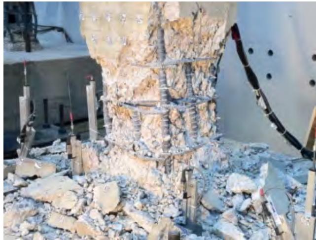
Figure 5.30 Concrete crushed, buckled longitudinal bars and opened ties in the corner of the column's bottom.
