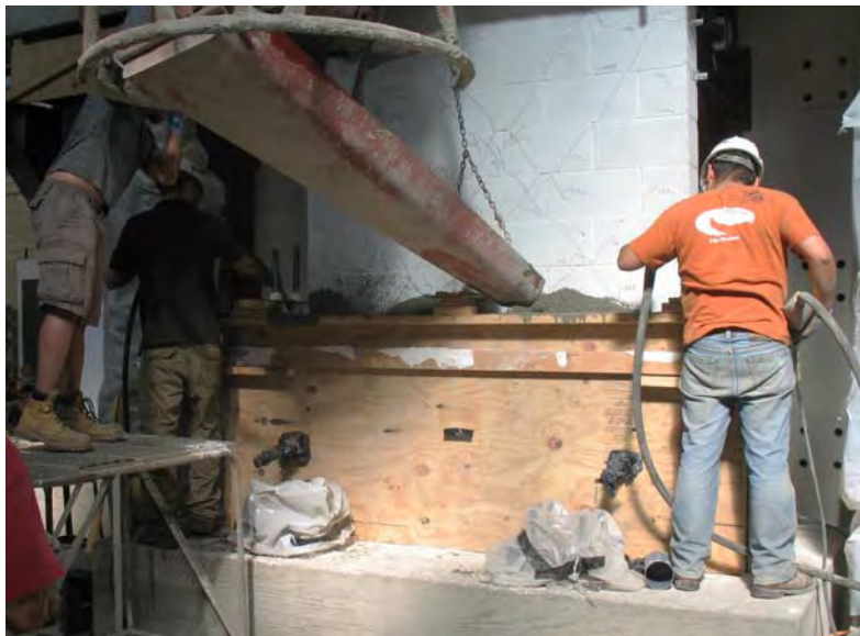
Figure 6.39 Casting of the concrete ring beam.
