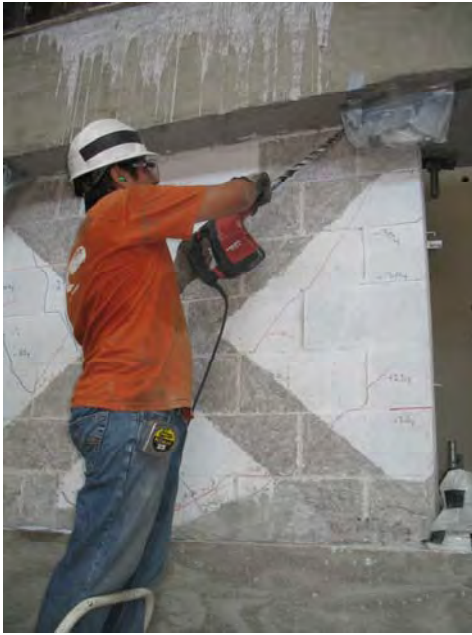
Figure D.8 Drilling the holes for CFRP anchor application (left) and drilled holes with rounded edges (right)
