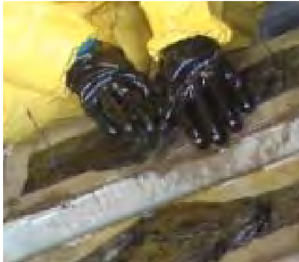
Figure 4.29 Application of the patch on the CFRP anchor
