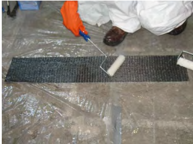
Figure D.20 Application of the epoxy on the strip for the CFRP U-patch
