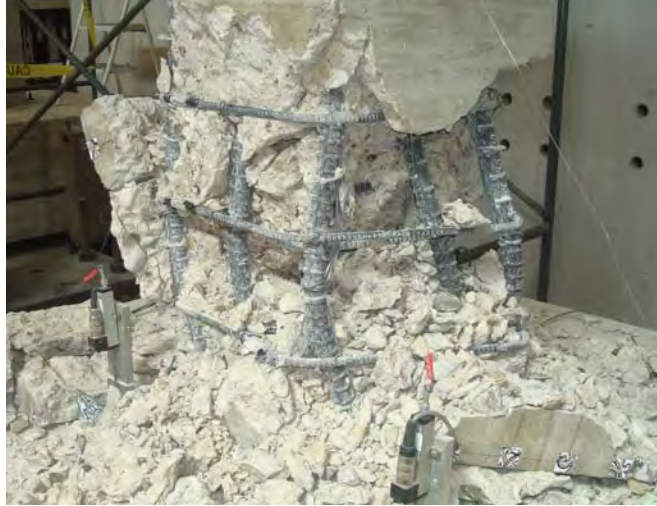
Figure 5.20 Concrete crushing, bars buckling, and opening of the transverse reinforcement at the bottom of column.
